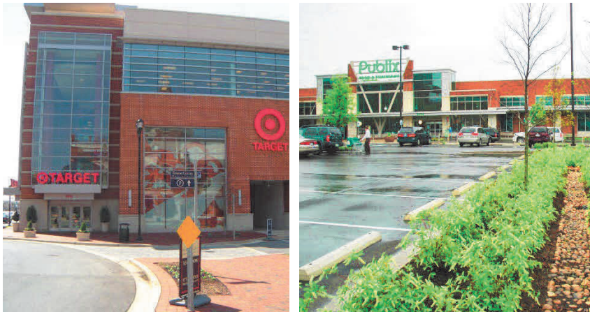
Figure 5.7.F(1): Examples of Large Retail Establishments
