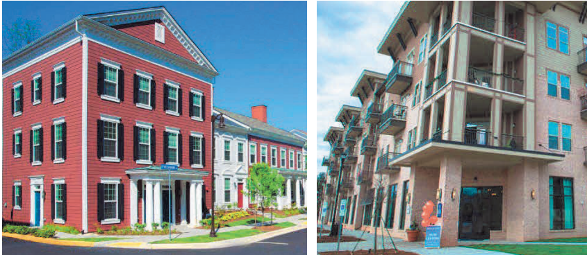
Figure 5.7.D(5)c: Examples of Front Façades
